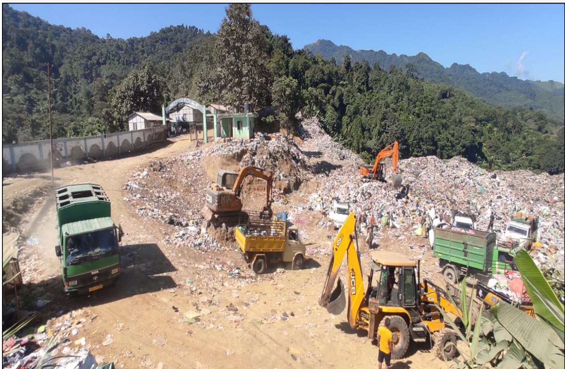
Entry Site and Stock point under operation for Segregation
